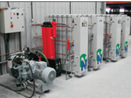
Using PSA gas generator and WP 4331 high-pressure 'H' series compressor
